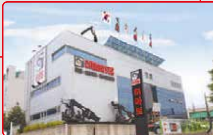
Cargotech Korea Co., Ltd. Metropolitan Area Center
